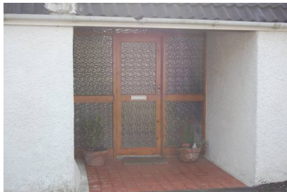
Inappropriate door replacement
