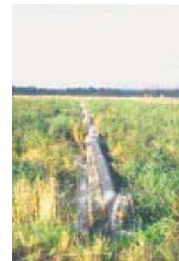
Treating sewage in reed beds at Valleyfield
