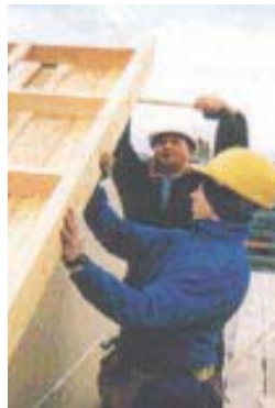
Kingdom Housing Association Development at Turner Crescent, Methil
